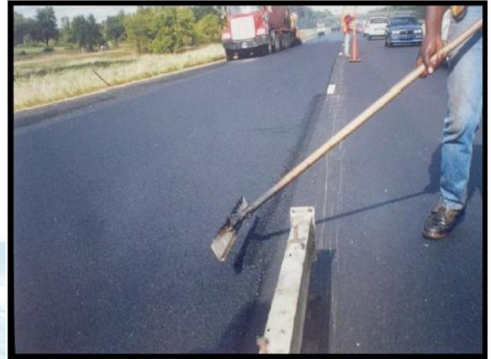
FIGURE 6 Luting of longitudinal joint.
