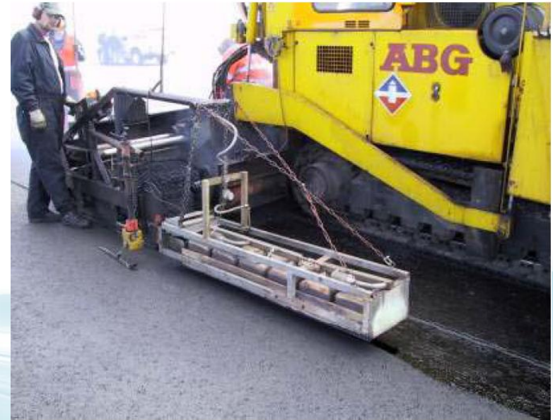
FIGURE 3 Use of joint heaters at longitudinal joints.
